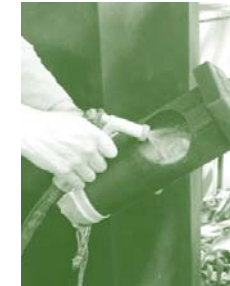
Invert the RiverSafe filter sock; clean with a hose
