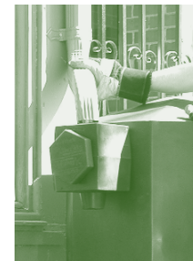
Check the downspout connections
