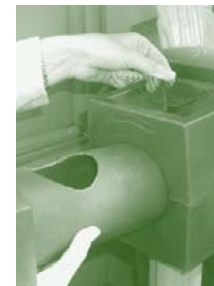
Inspect the filters
