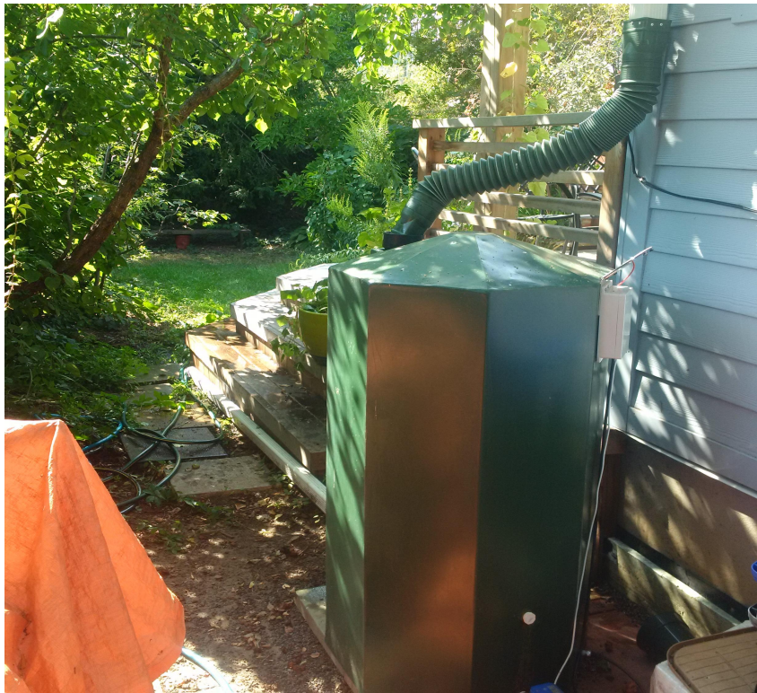
Figure 1.1: Installation of ARB system on Hampton Ave.
