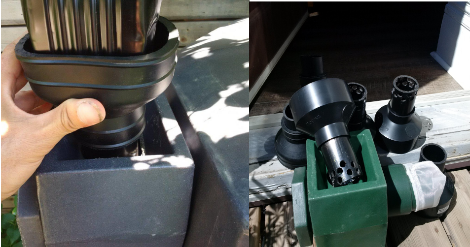
Figure 1.2: LEFT: Storm funnel (black) in diverter box (grey). RIGHT: Uninstalled storm funnels (black) and diverter box (green) with filter (white).
