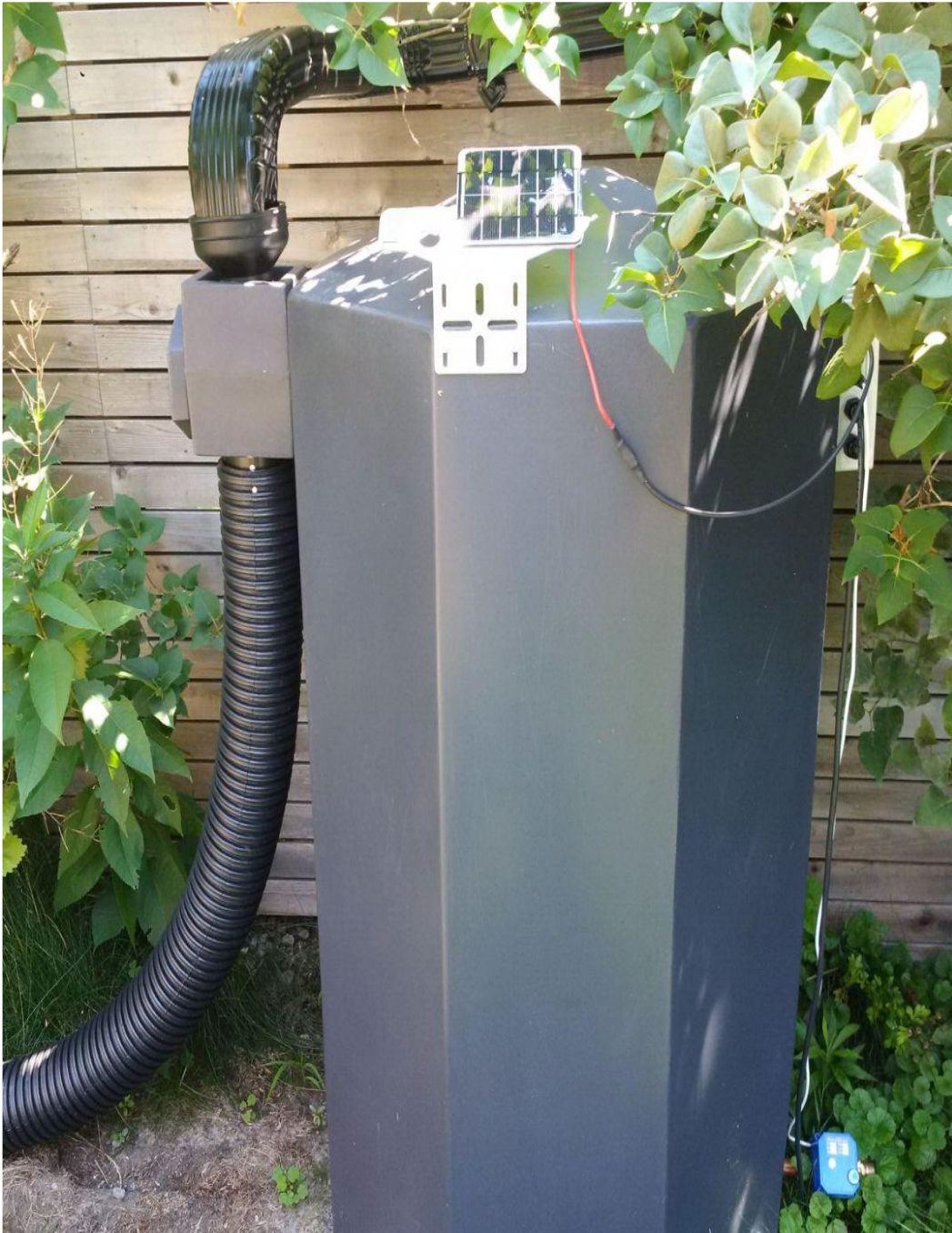
Figure 1.1: Shows a fully installed rain barrel
