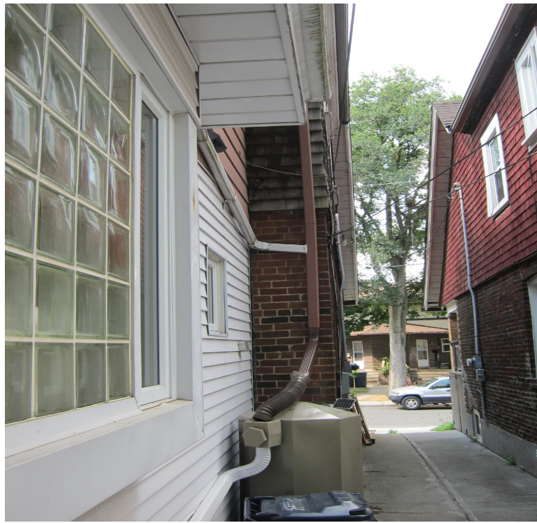
Figure 4.3: North-facing view of Cavell Ave. fully installed ARB system, with downspout disconnected from the storm sewer and overflow and bypass running along house to French drain (not pictured).
