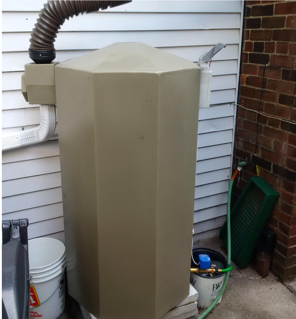
Figure 4.1: Installed Cavell Ave. ARB system with solar panel (right) and storm funnel attachment (left).
