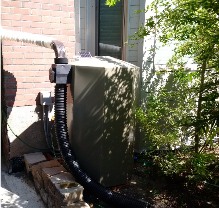
Figure 5.2: Installed ARB system at Withrow Ave., with storm funnel attachment (to the left) and solar panel (at the back).
