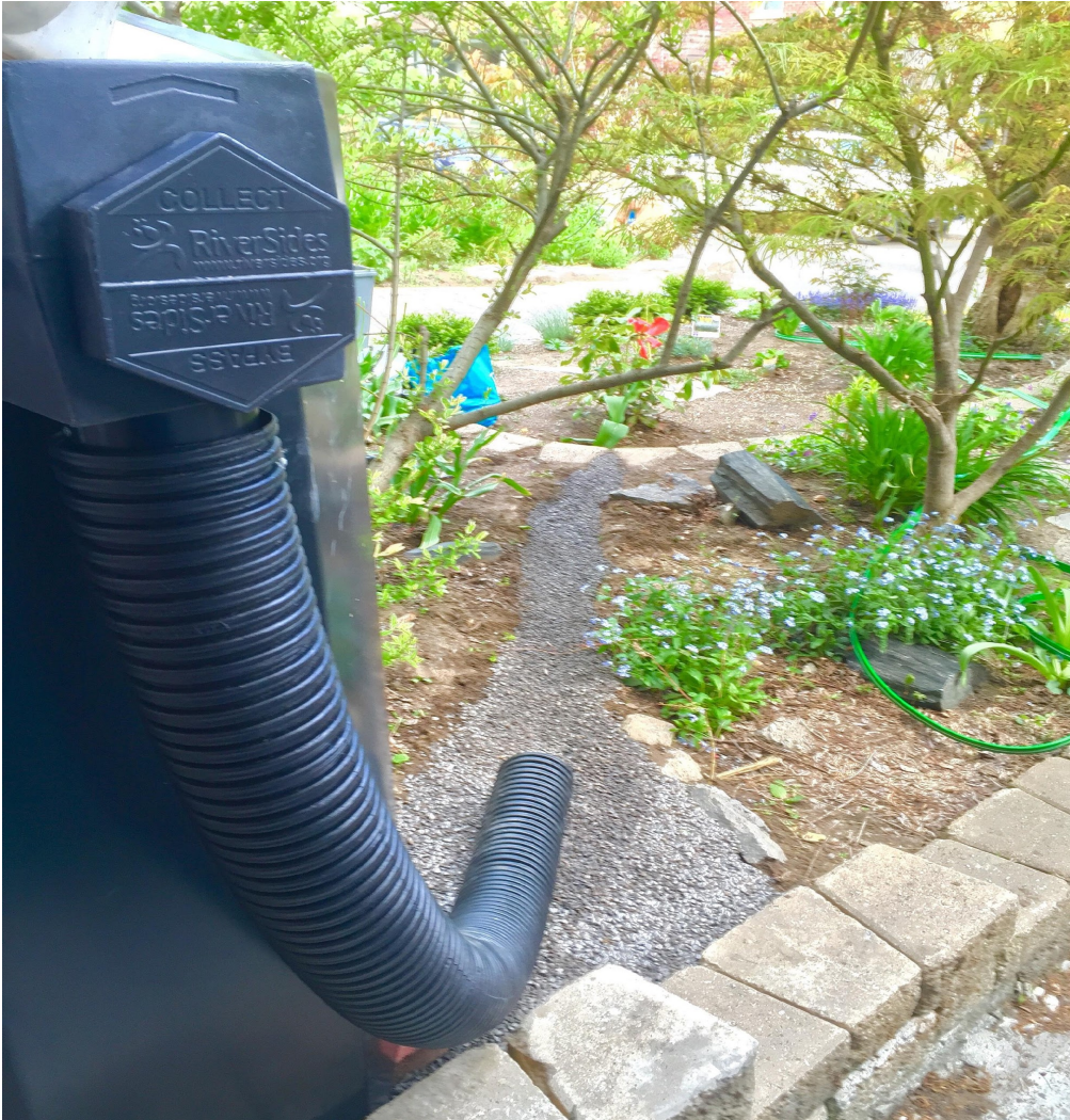
Figure 5.1: Rain barrel diverter and bypass flowing to rain garden on Withrow Ave.
